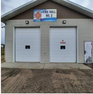
Front Bay Doors
