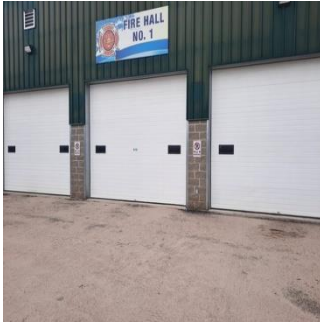
Front Bay Doors
