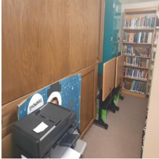
Library Electrical Panel Area
